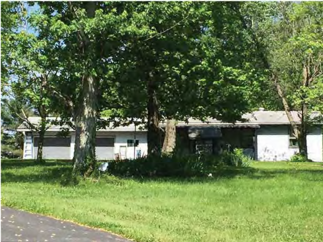
12. NC 5097 N Old SR 37, modest ranch with new garage doors, some new windows, vinyl
