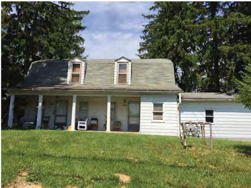
22. IHSSI 105-055-20031 (C) 4871-4869 N Old SR 37, new windows, siding, doors (NC)
