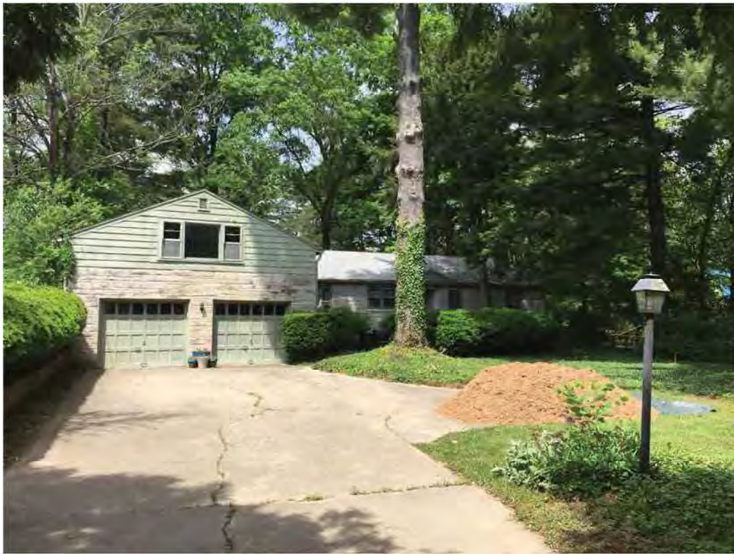
31. IHSSI 105-055-20036 (C) 4393 N Old SR 37, c. 1951 large ranch with integrity, original windows, garage doors, clapboard
