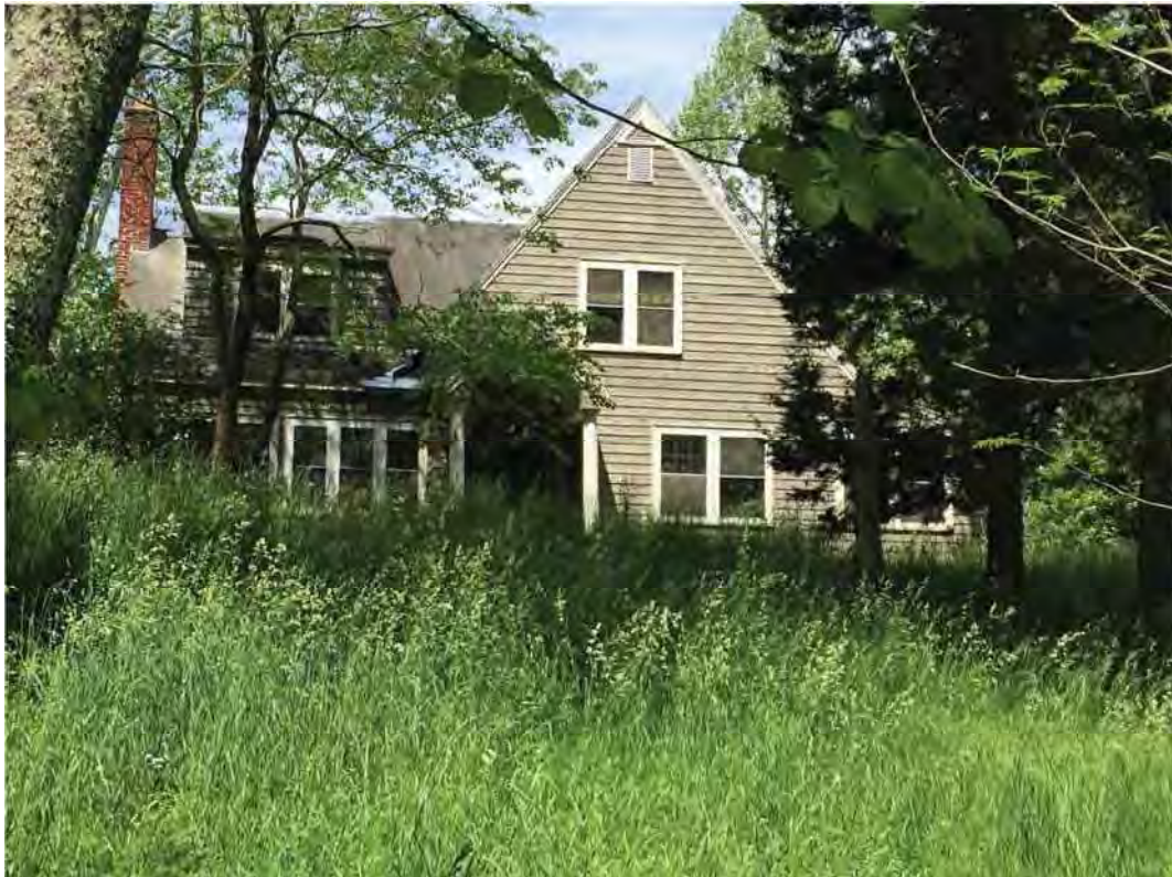
24. IHSSI 105-055-20037 (C) 4425 N Old SR 37--enclosed porch on north side (behind tree), additions on north side & rear
