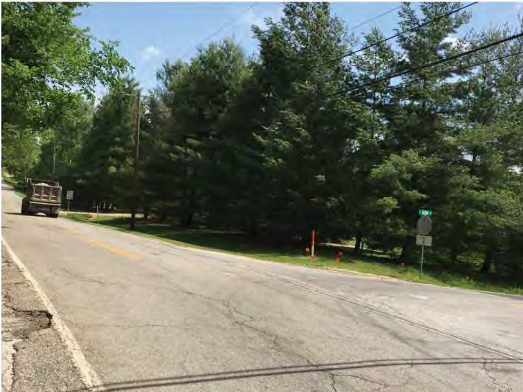
28. Looking north at N Old SR 37 near Bethel Road
