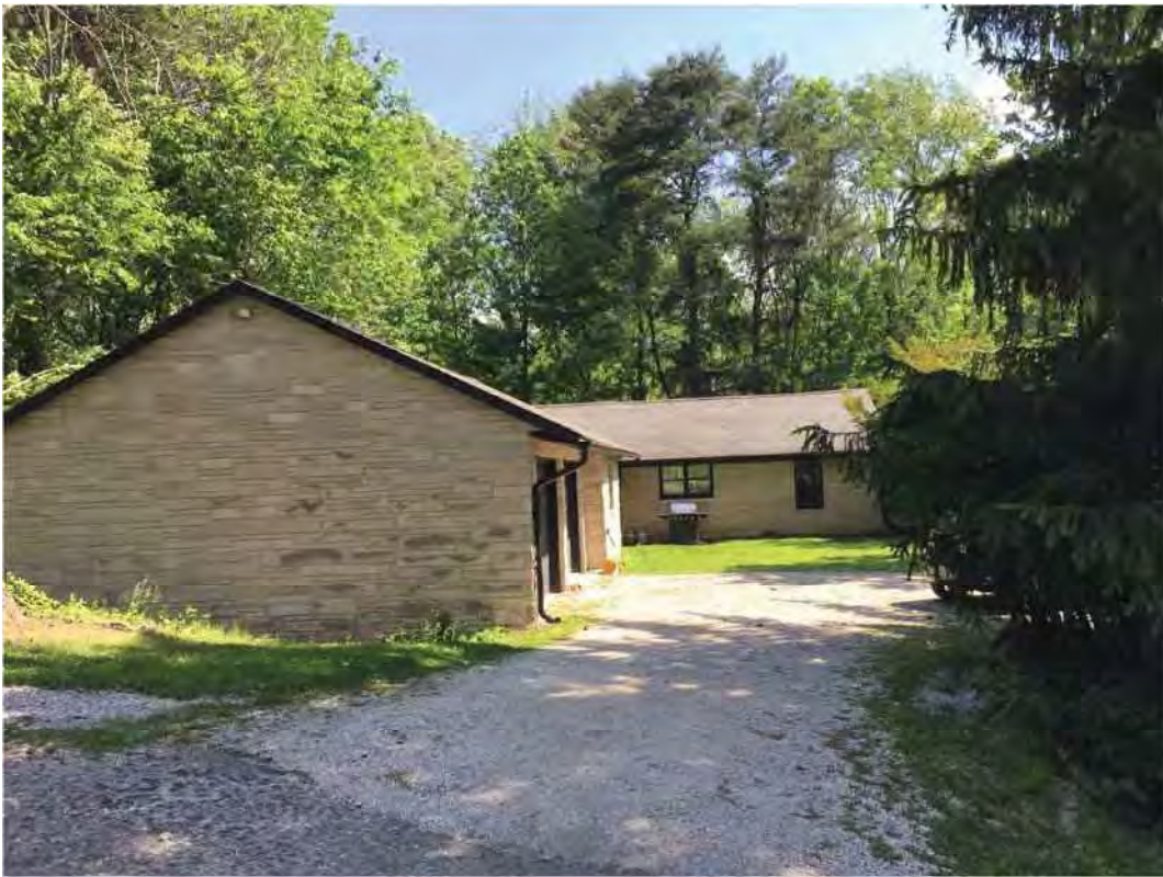
11. IHSSI 105-055-20076 (C) 5169 N Old SR 37, stone-veneer ranch with large garage addition
