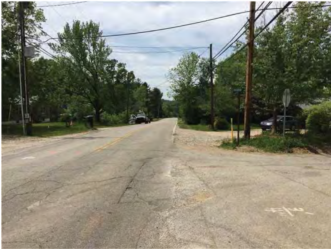
35. Looking north at N Old SR 37 from end of APE
