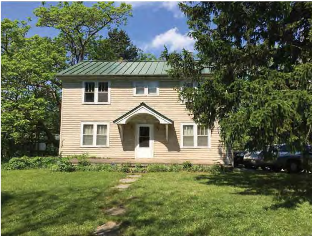
13. IHSSI 105-055-20075 (C), 4899 N Old SR 37, altered double-pile, vinyl siding, porch canopy and new windows added c. 1920s
