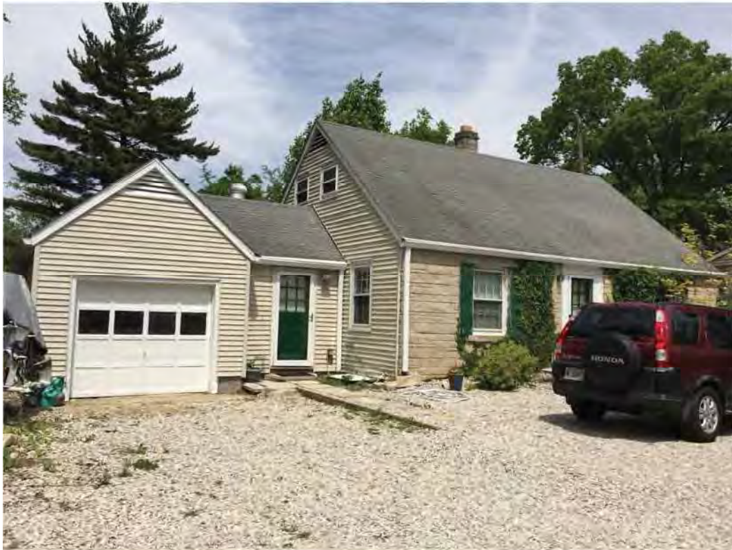
36. IHSSI 105-055-20039 (C) 4293 N Old SR 37, cottage with attached garage addition, original windows, vinyl siding
