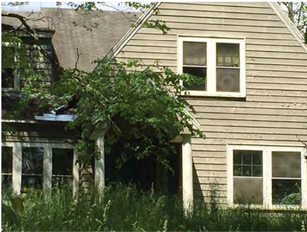
25. IHSS 105-055-20037 close up showing clapboard siding, original windows
