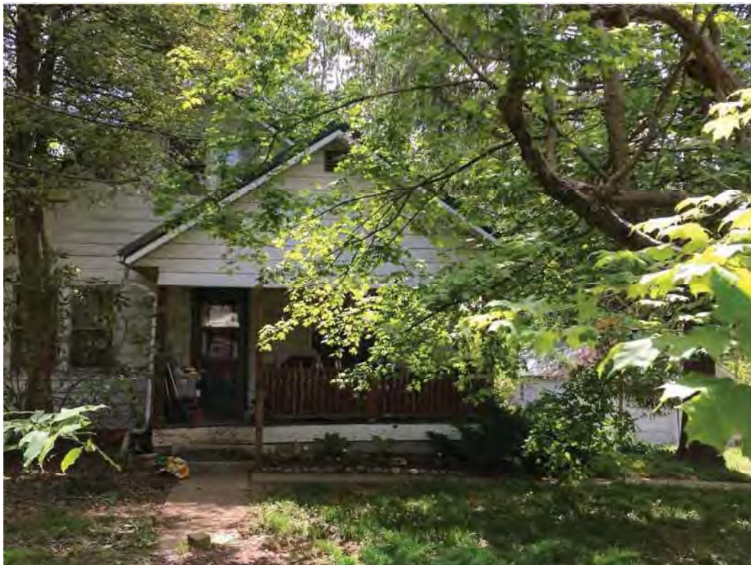
32. 105-055-G9 (C) 4328 N Old SR 37, double-gable with new porch baluster
