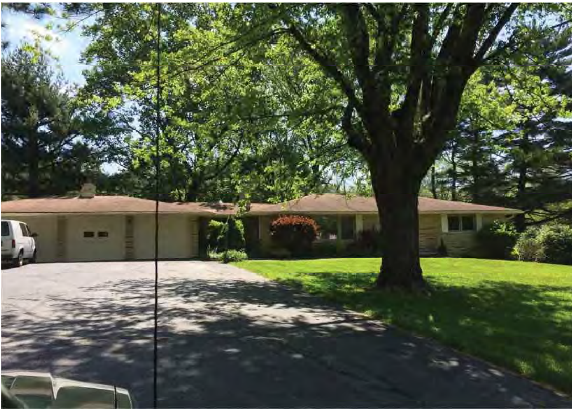
17. 105-055-G6 (C) 4850 N Old SR 37, two-section massed ranch with breezeway and dovecote on garage, high integrity, but replaced garage doors
