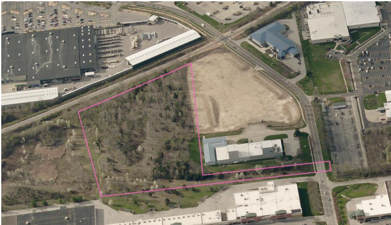
Figure 2. Pictometry photo from April 2020, looking south.
