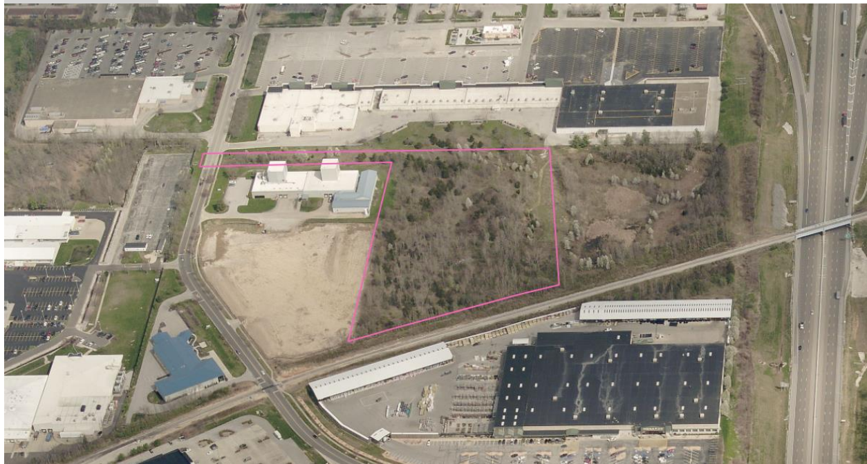
Figure 1. Pictometry photo from April 2020, looking north.
