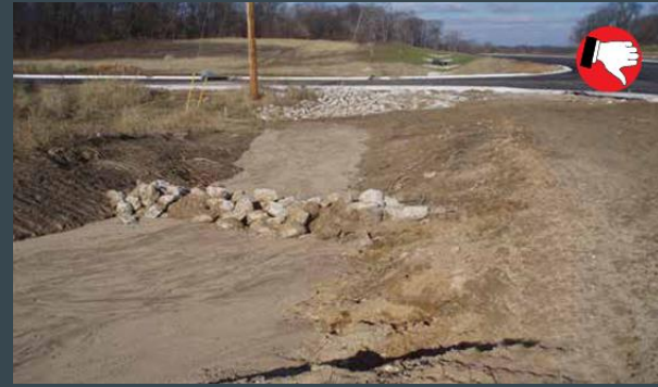
Rock check dam not built to specification. Not shaped correctly, no filter stone, no geotextile. The check dam should be rebuilt.
