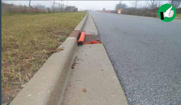
Inlet bag protection can be used on curb inlets with active traffic. Maintain bags after each storm event. Bags can get heavy and hard to maintain when very full.
