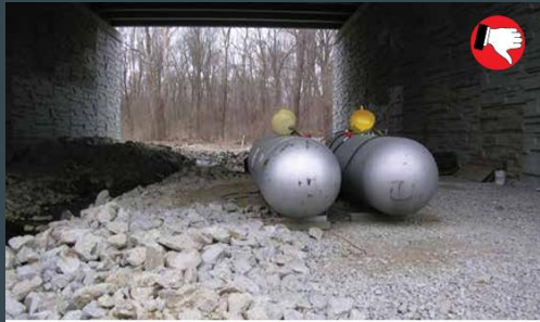
Locate fueling operations, temporary toilets and staging away from waterways and other hot spots.
