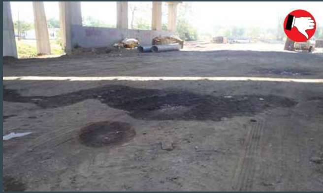
Prevent fuel or other toxic spills. Locate spill cleanup kits in accessible areas and clean up immediately.
