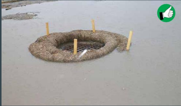
Filter sock inlet protection staked correctly.
