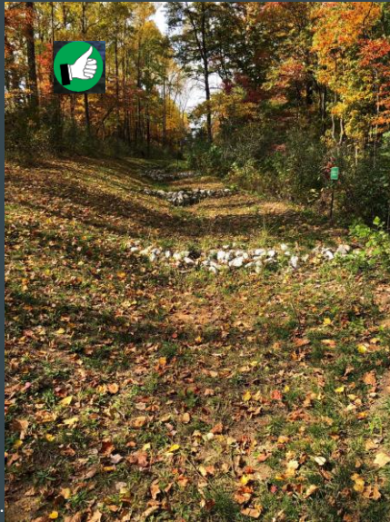
Rock check dam not built to specification. Not shaped correctly, no filter stone, no geotextile. The check dam should be rebuilt.
