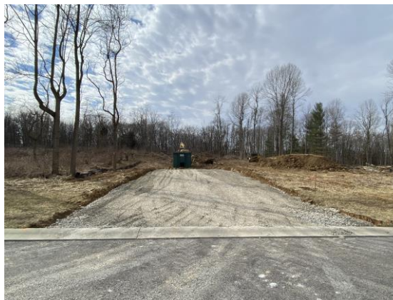
Maintain proper stone base for duration of project.
