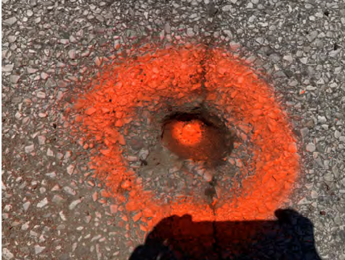
Photo Orientation & Description: Wash_M15 from above
