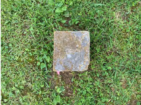
Photo Orientation & Description: Per_A17 from above
