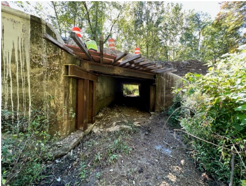
STR #3 repair (false work)
