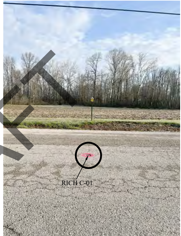
Looking North at RICH C-01
