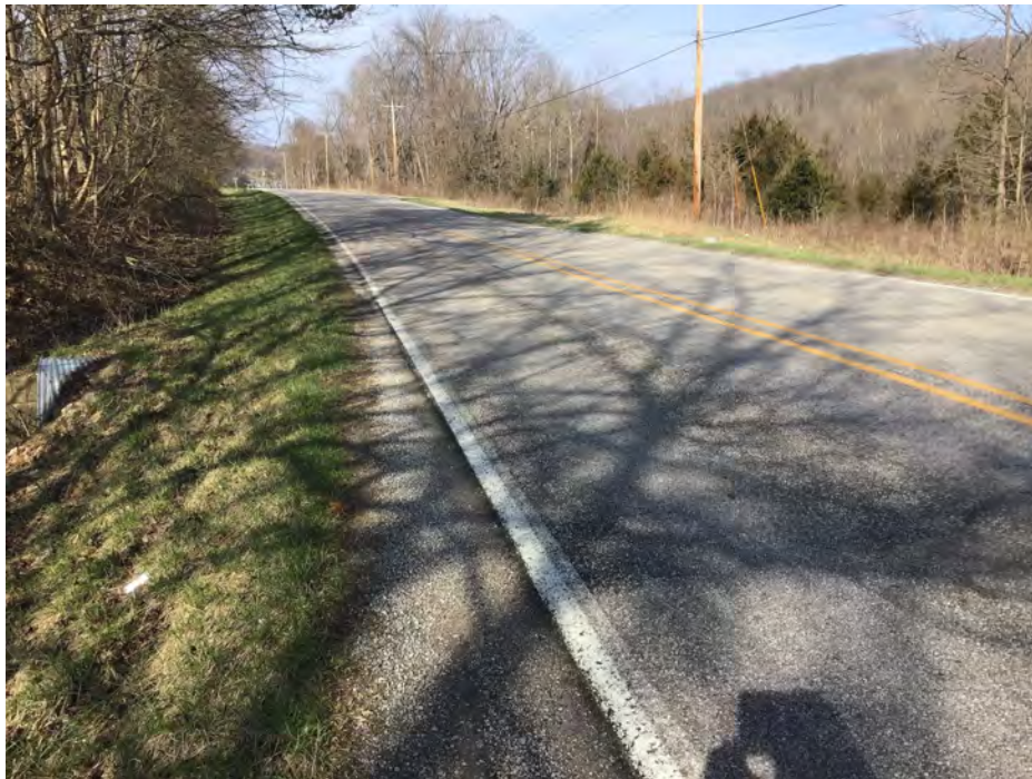
PHOTO 2 Condition Description Roadway facing West
