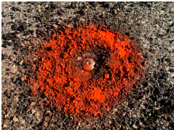
Photo Orientation & Description: Mag spike set over rebar at A11
