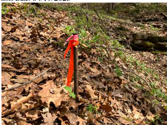
Photo Orientation & Description: Forming pin at E09
