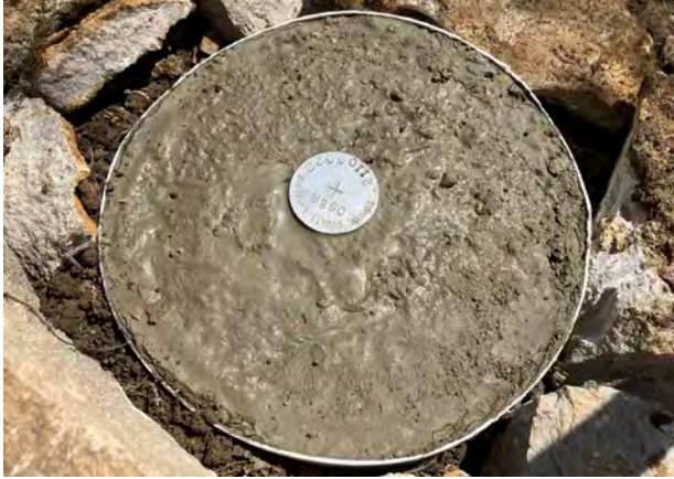
Photo Orientation & Description: Capped rebar in concrete
