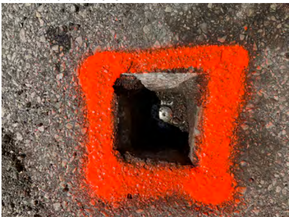
Photo Orientation & Description: Magspike at E01
