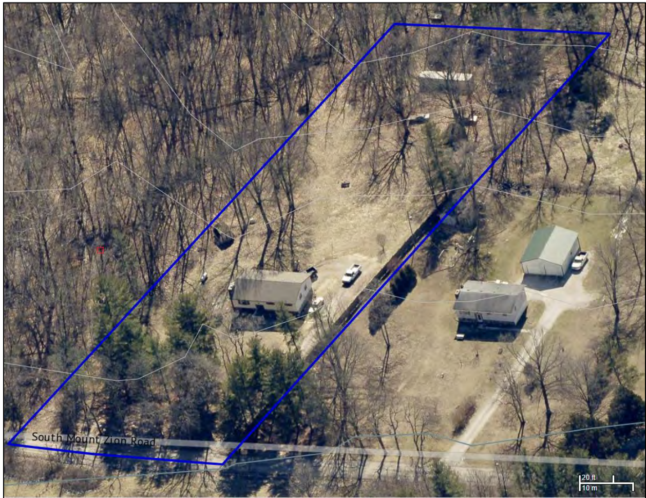
Photo 2: Aerial view of petition site from the south (2022)
