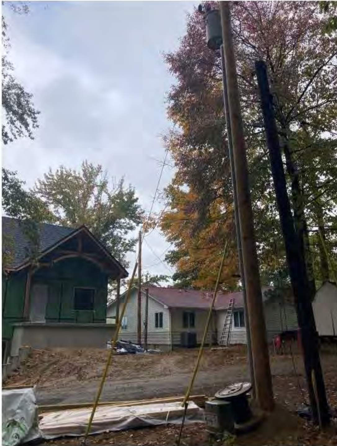
Utility poles recently replaced
