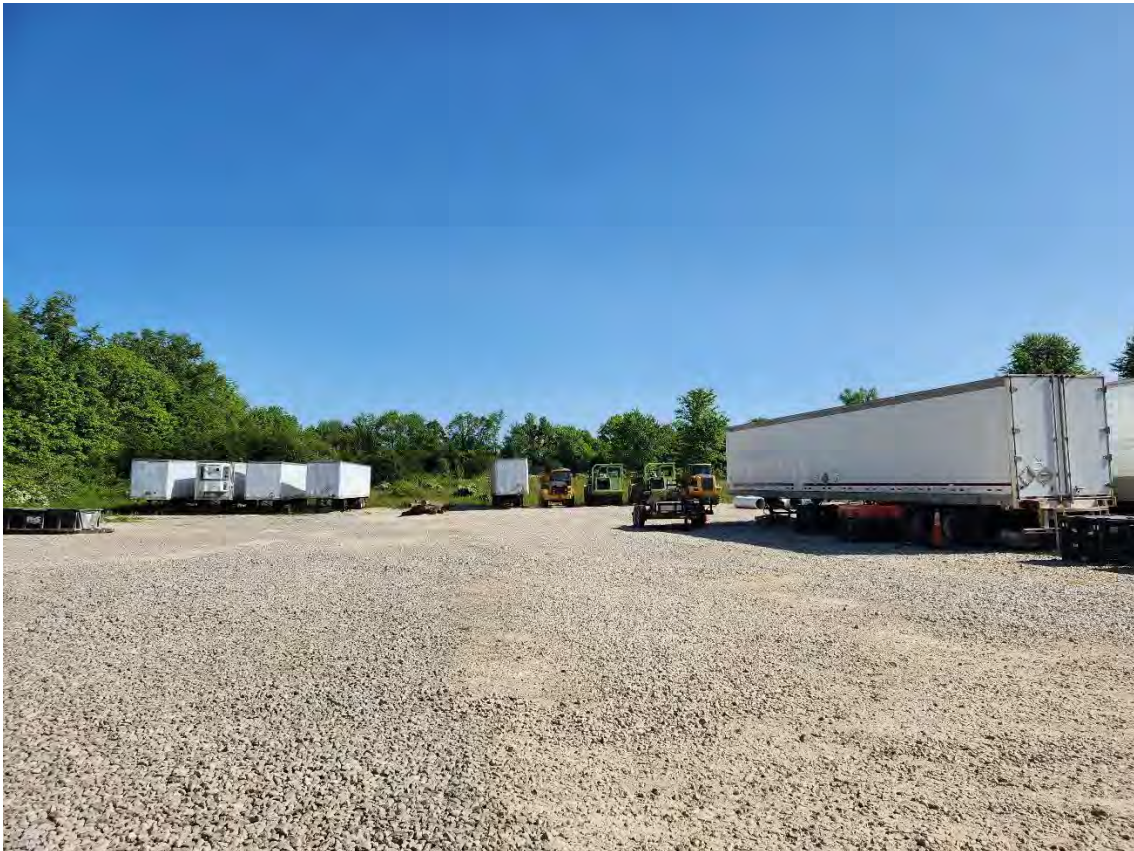
Photo 4. Site of Sinkhole 'A' (Facing North)
