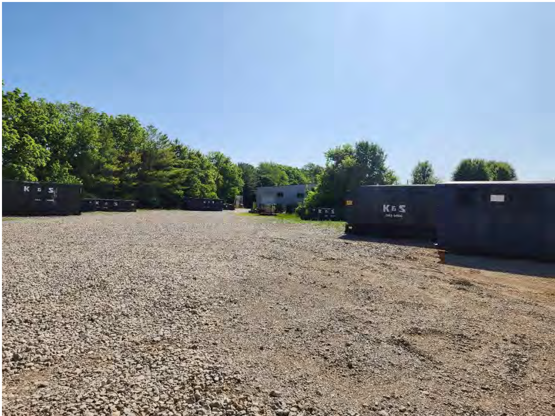
Photo 5. Site of Sinkhole 'B' (Facing East)
