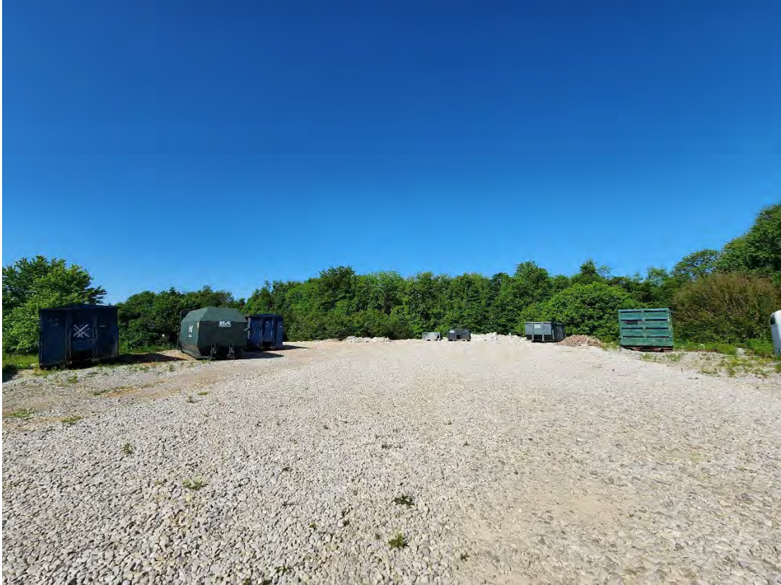
Photo 5. Site of Sinkhole 'B' (Facing West)
