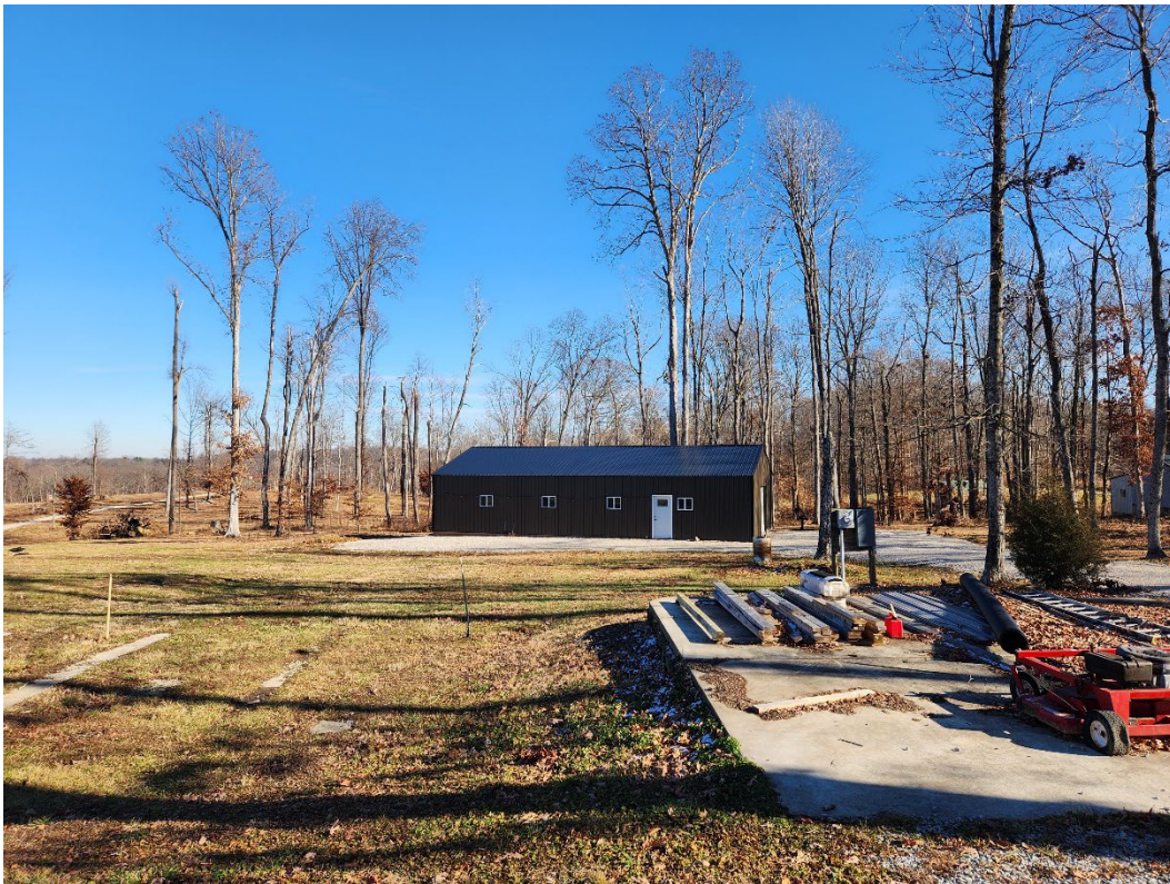
Photo 3 – Facing East (storage structure)
