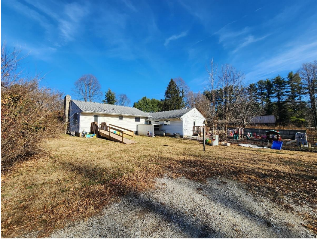
Above: A view of the principal use structure from the rear
