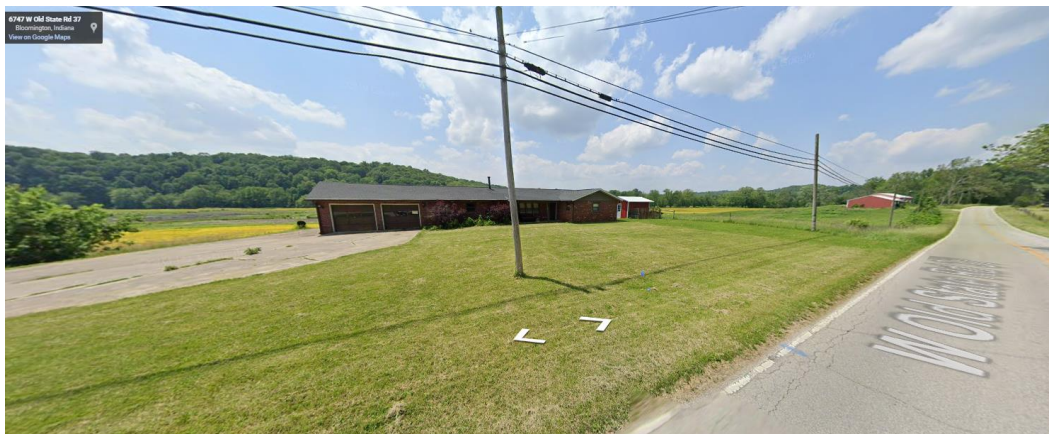
Image 1: Existing Residence and Agricultural Structure
