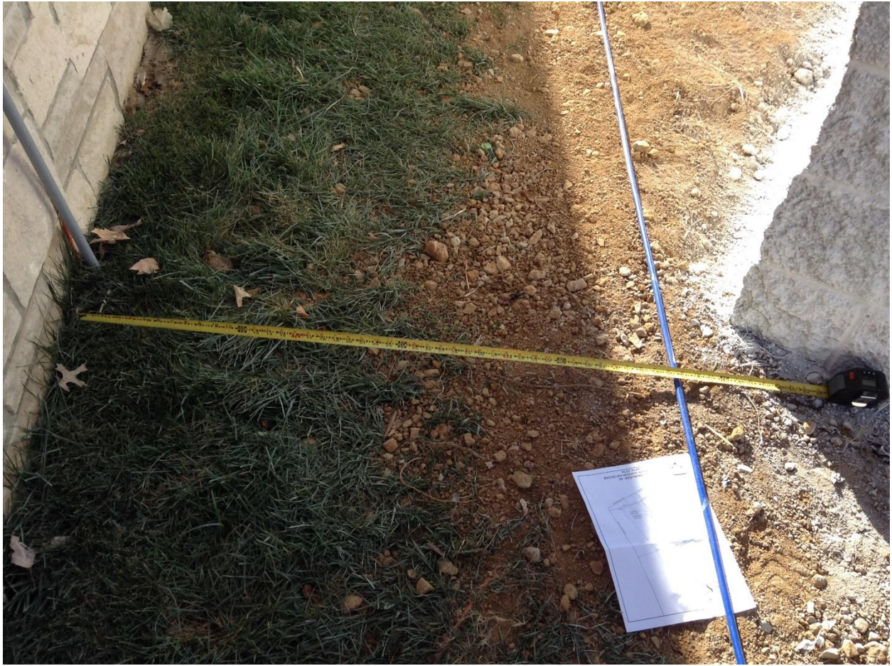
Site Photo 2: Staff measurement
