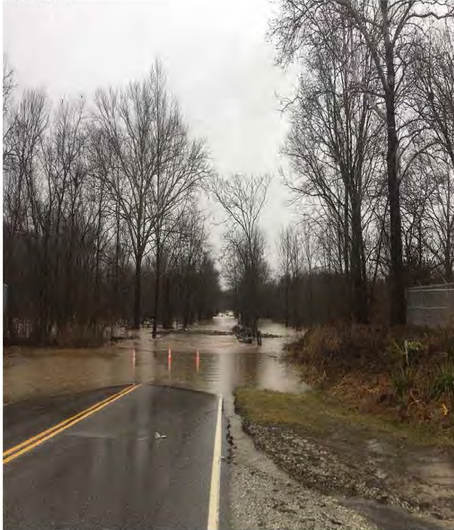
2-7-19. Looking north on Rogers Street at S.R. 37. Clear Creek is on the left, Jackson Creek is in the foreground, just past the traffic cones.
