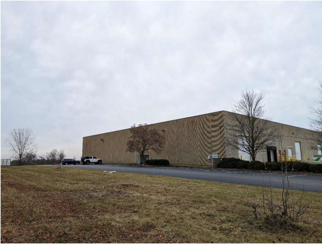
Photo 6: Petition site and adjacent business – facing southeast
