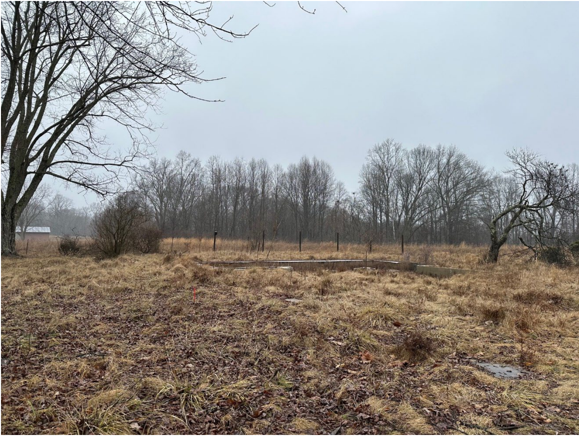
Photo 3: The foundation of a demolished home.
