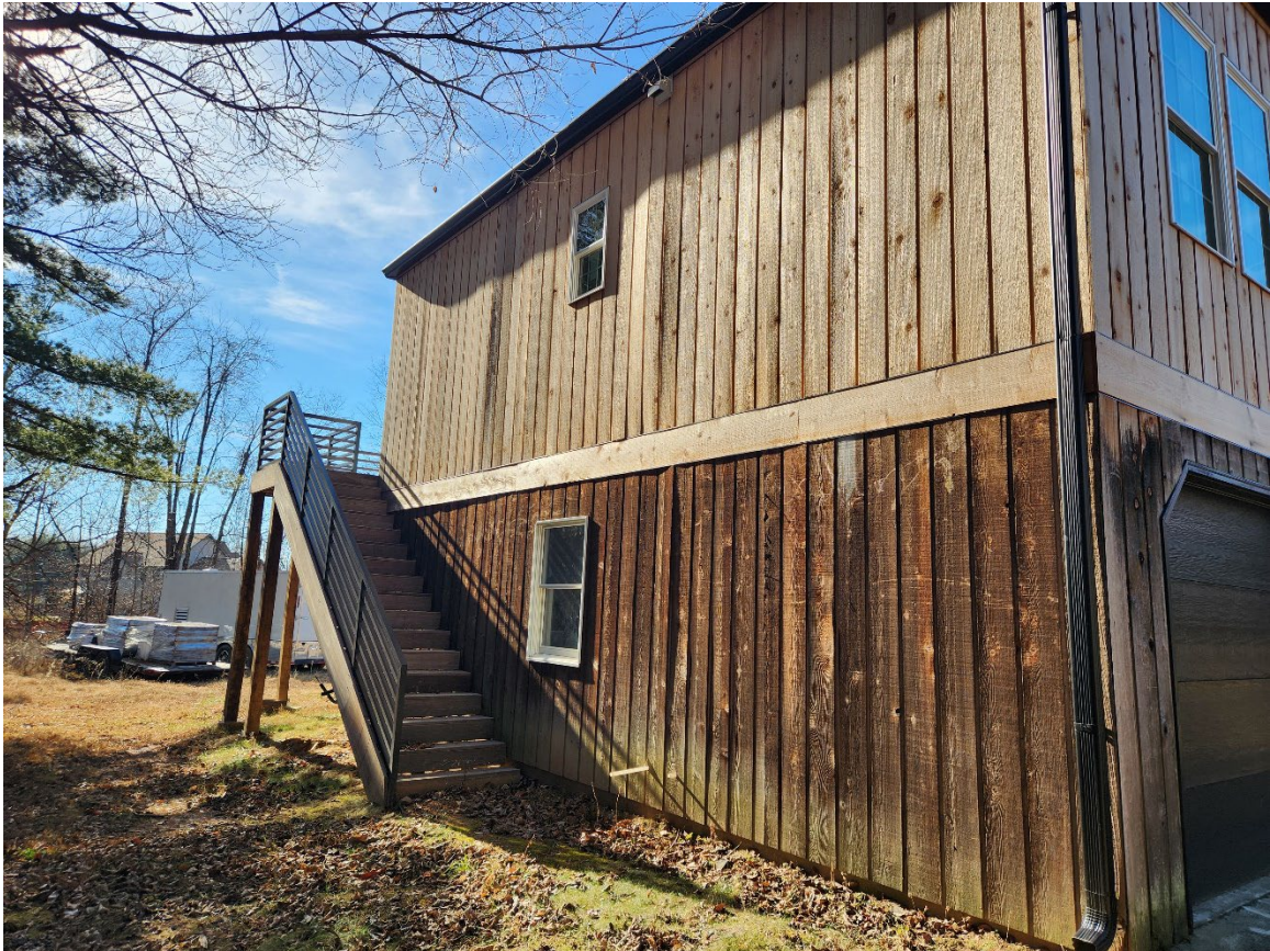
Photo 4 – Facing Southwest (east side of structure)
