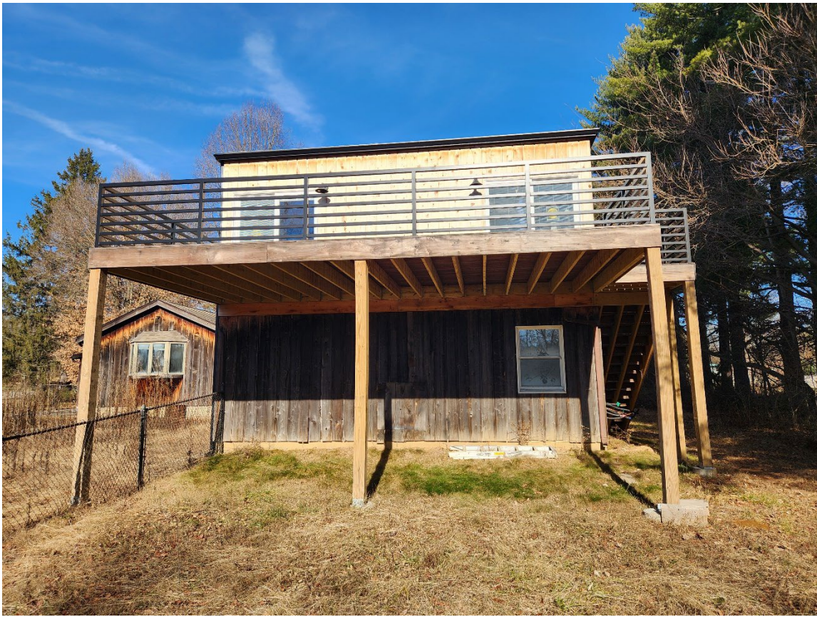
Photo 5 – Facing North (rear side of structure)
