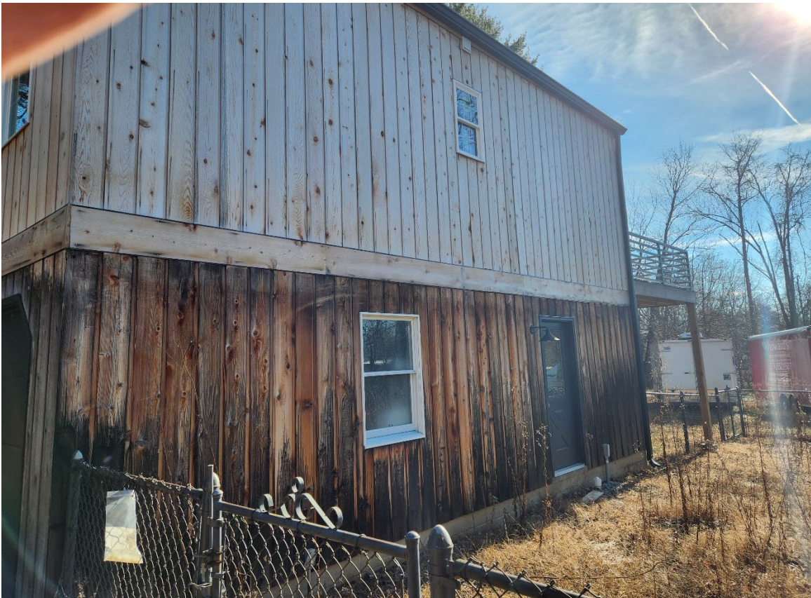
Photo 6 – Facing Southeast (west side of structure)
