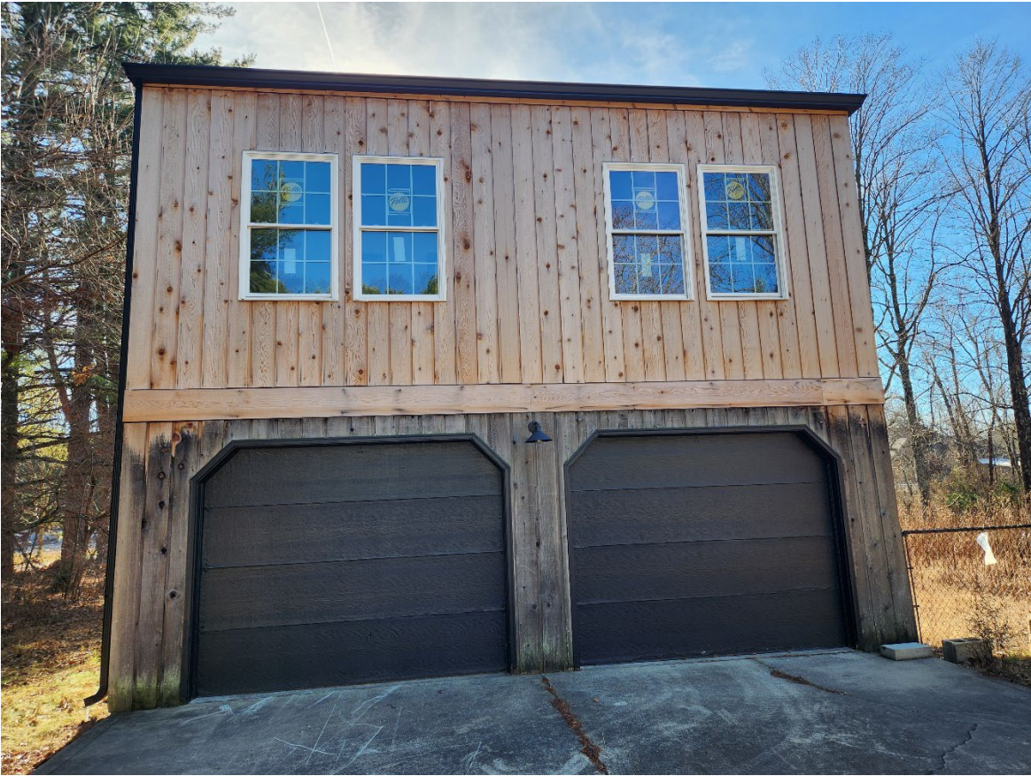
Photo 3 – Facing South (front of structure)
