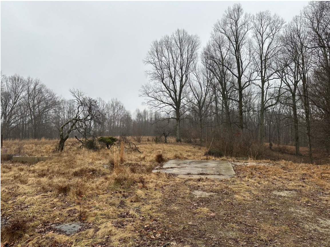
Photo 4: The foundation of a demolished garage.
