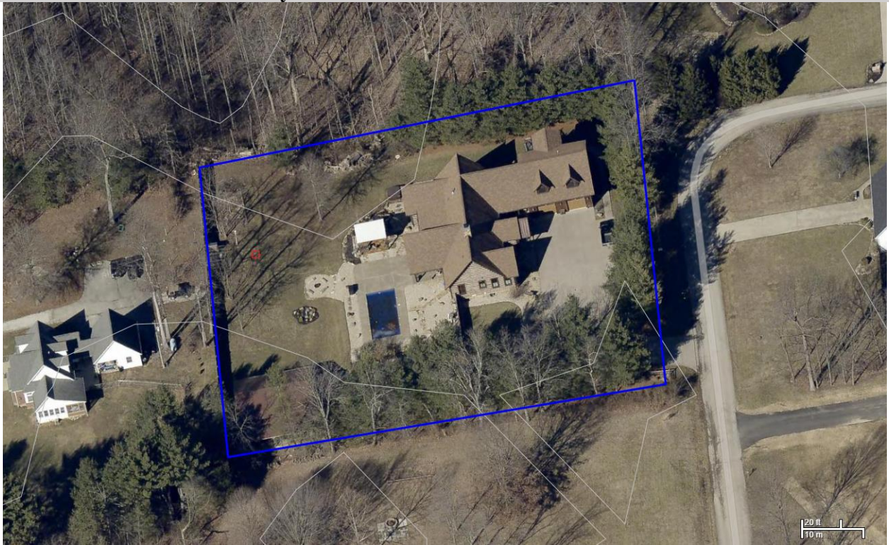
Photo 1 – view from South
