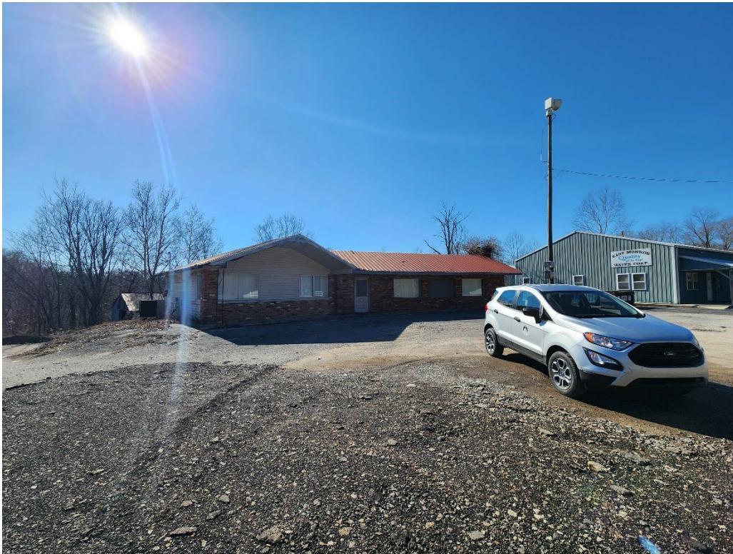
Photo 1 – Facing Southwest (parking lot/primary structure)
