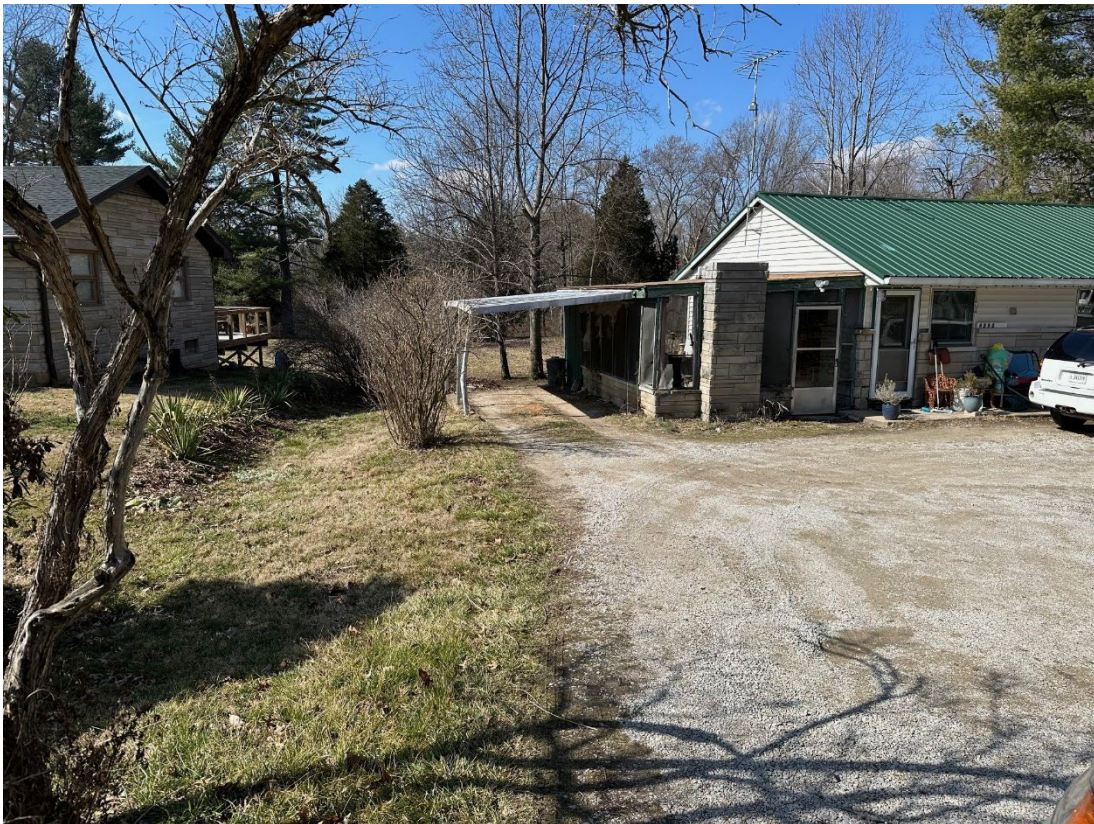
Photo 4: View of the existing canopy and section of the home to be replaced by the garage.
