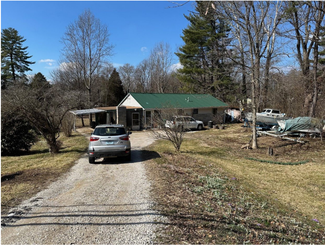
Photo 3: View of the property from the right-of-way.
