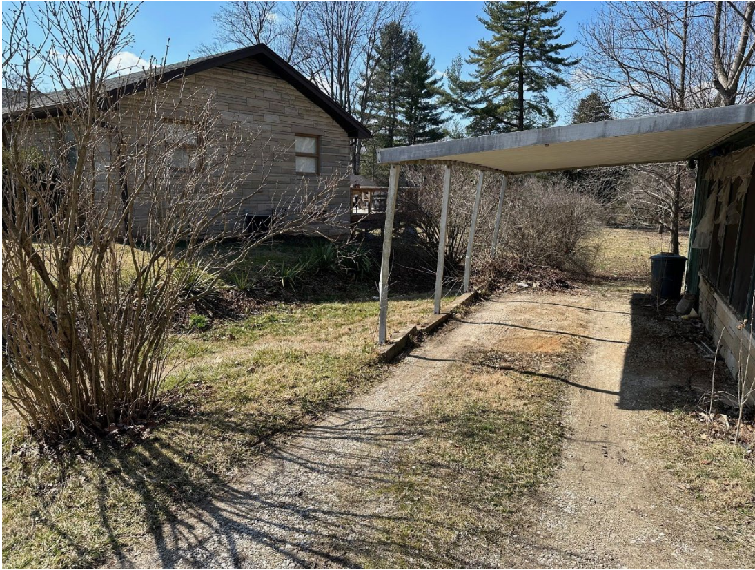
Photo 5: View of the existing canopy and proximity to side property line
