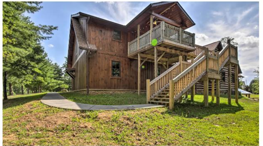
Exterior | Homeowner On-Site
