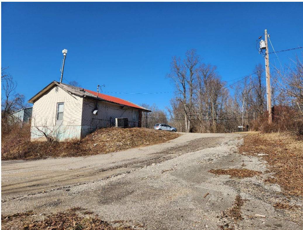
Photo 4 – Facing Northwest (view from existing driveway towards the front of the property)
