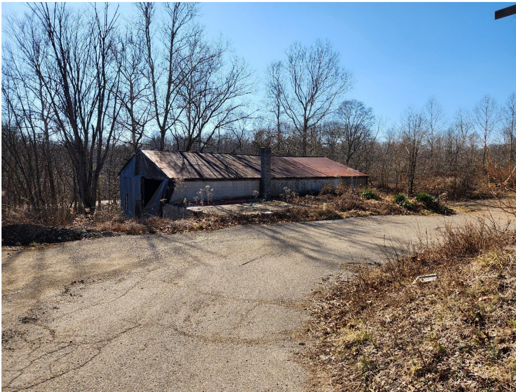
Photo 5 – Facing Southwest (second structure located in the rear of the property)
