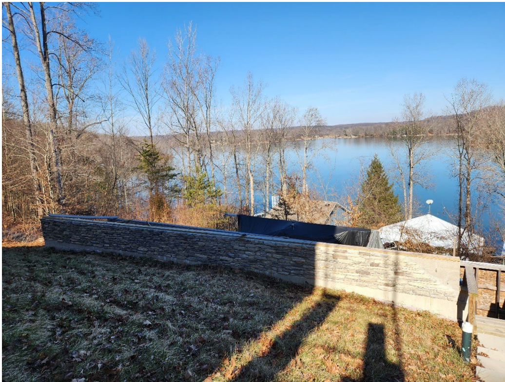
Photo 6 – Facing North (the top of the structure)
