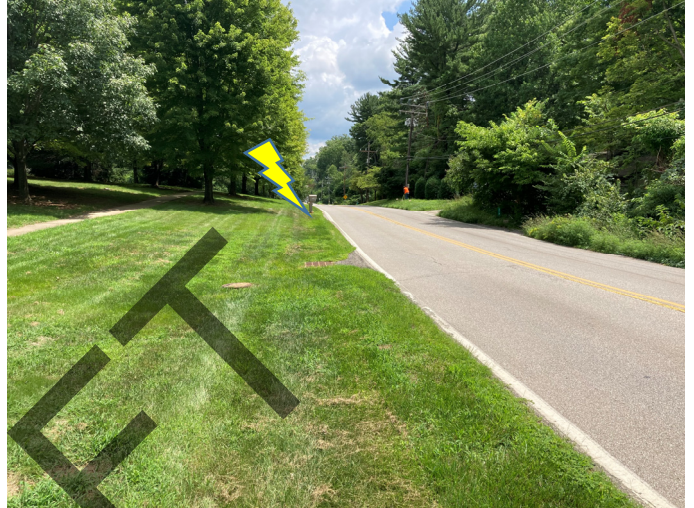
Photo Orientation & Description: Looking east at Per_S05
