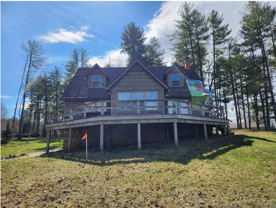
Photo 4 – Facing South (Back Deck)
