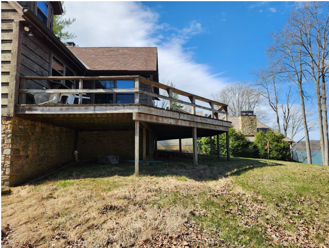
Photo 6 – Facing West (East side of deck)
