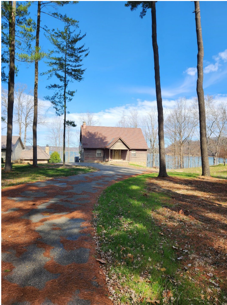
Photo 3 – Facing North (Primary Residence)
