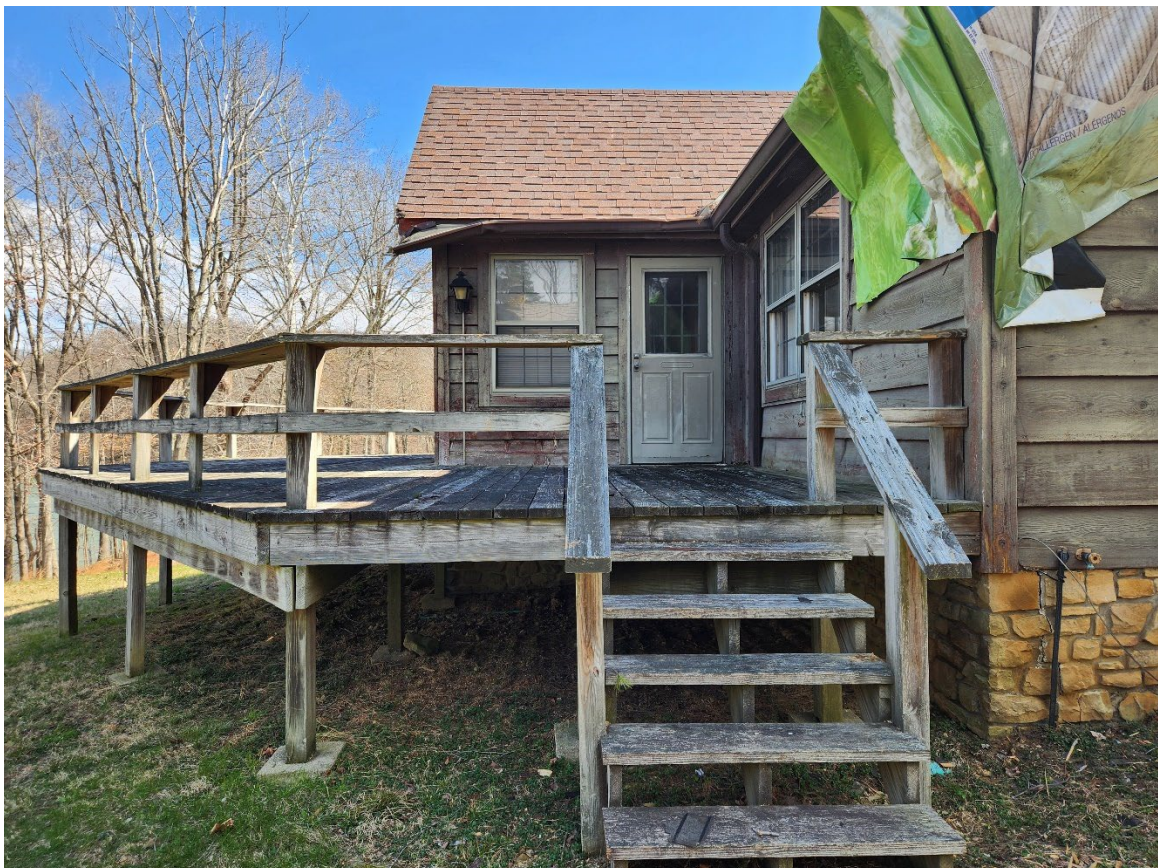
Photo 5 – Facing East (West side of deck)
