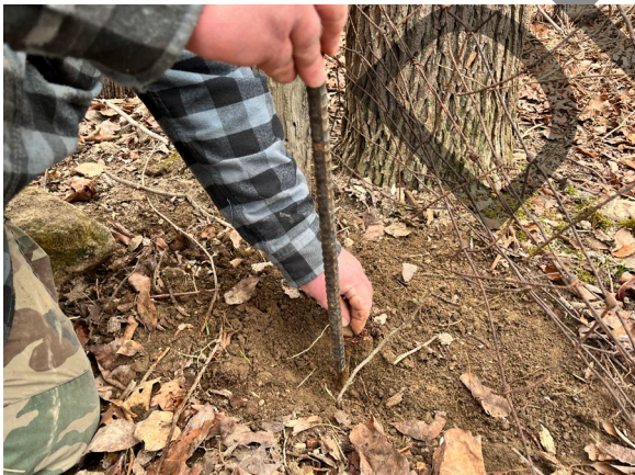
Photo Orientation & Description: From above, showing nail removed and rebar set in its former location.
