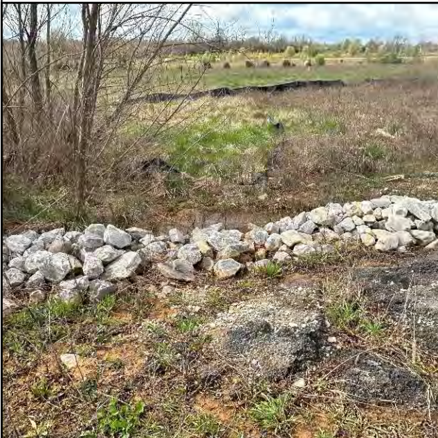
Photo 7: Riprap and silt fencing in vicinity of soil stockpile; View to the south
