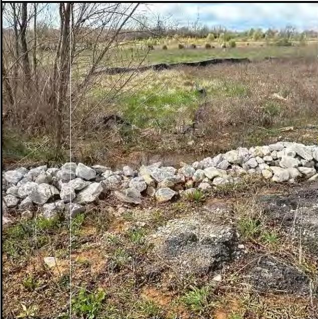
Photo 7: Riprap and silt fencing in vicinity of soil stockpile; View to the south
