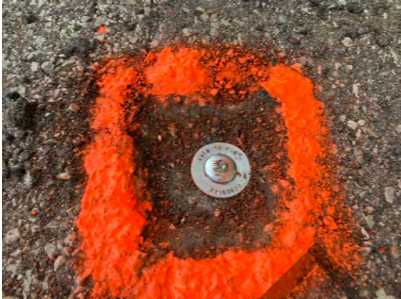
Photo Orientation & Description: Magspike at E19 from above
