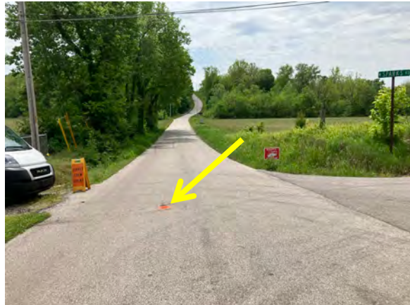
Photo Orientation & Description: Looking south at E23
