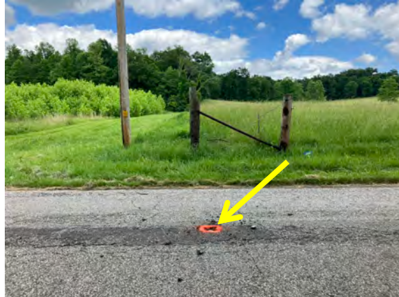
Photo Orientation & Description: Looking east at E19
