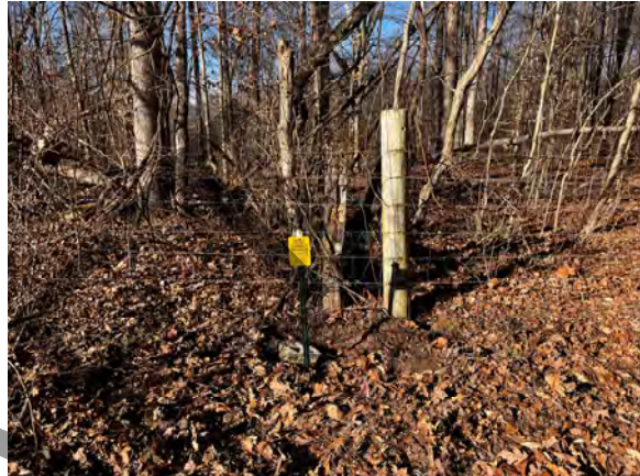
Photo Orientation & Description: From East looking West
