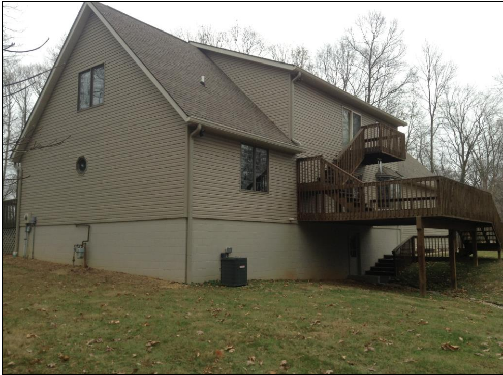
Figure 9. Facing northeast: view of the residence.
