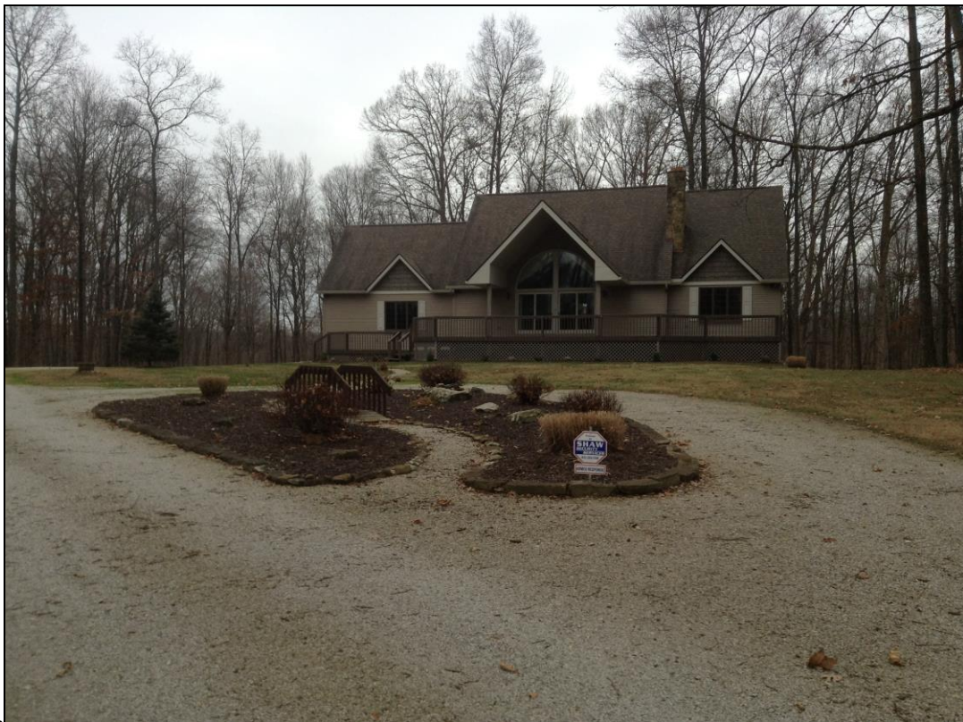
Figure 4. Facing south: view of circular drive and primary residence.
