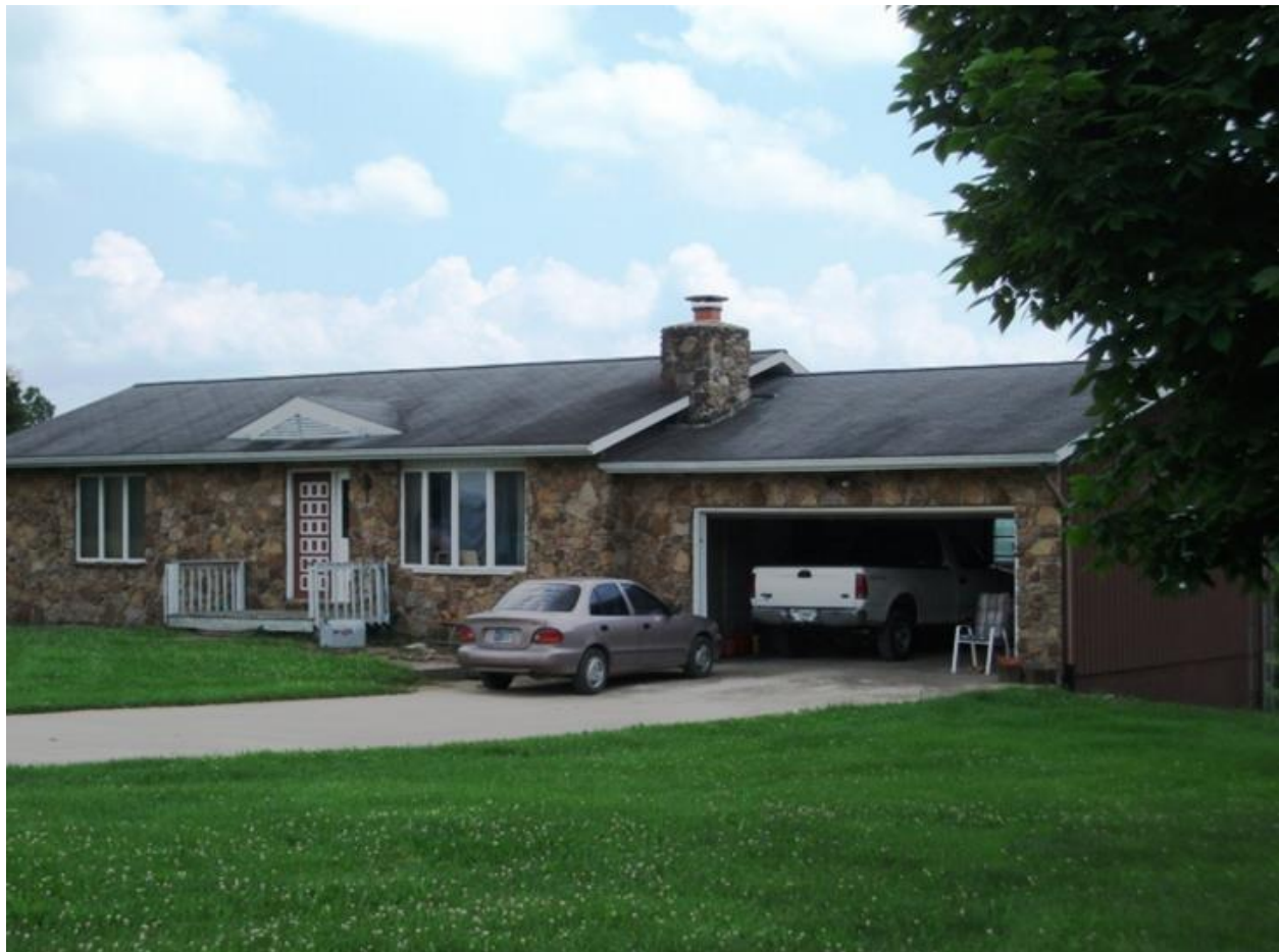
Figure 6. Facing southeast; existing home.
