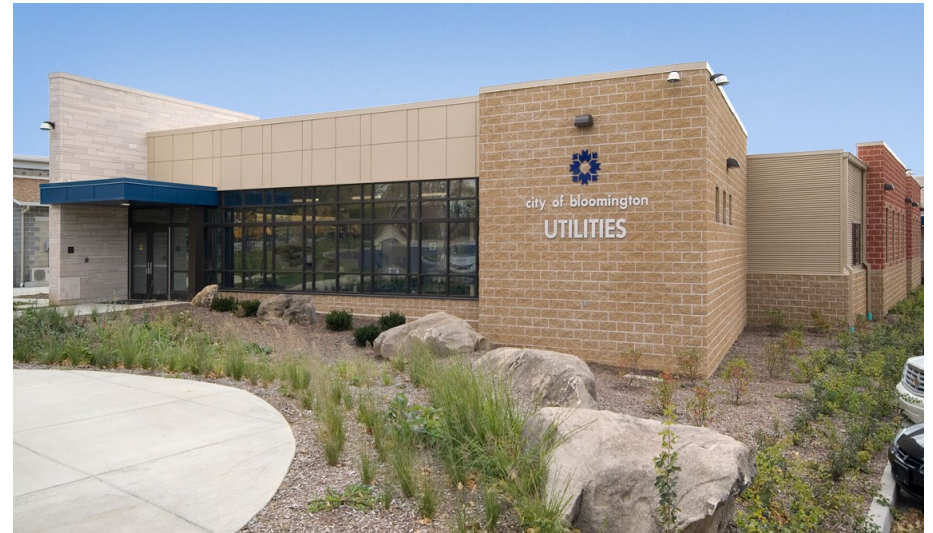
Bloomington Utilities Building
