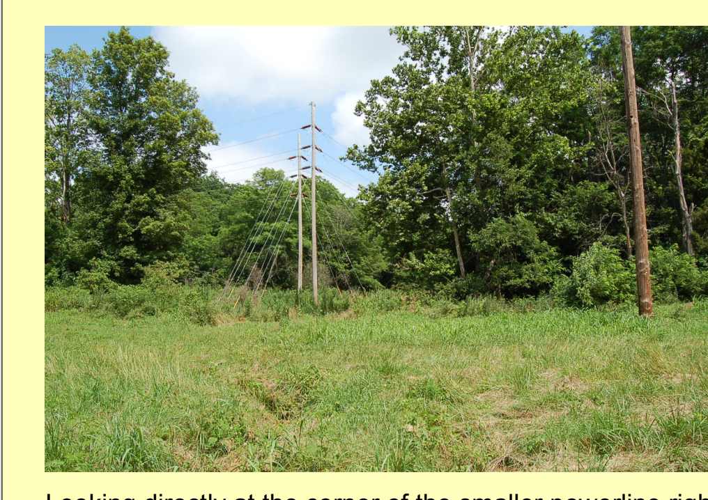
Looking directly at the corner of the smaller powerline right of way.
