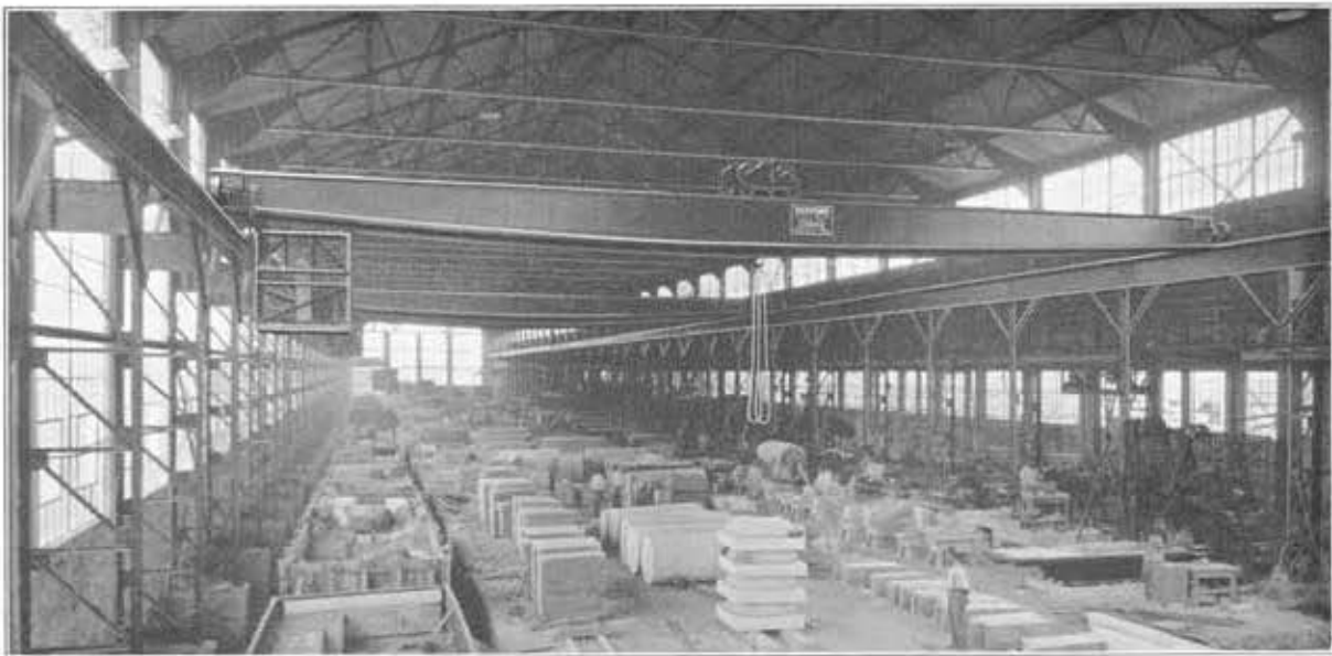
Consolidated Stone Company, Bedford, Indiana, showing 3-7½-ton 70' 0" span; 2-30-ton 70' 0" span three- and four-motor Cranes
