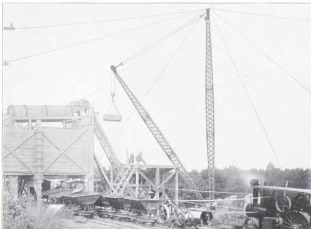
10-ton Bedford Steel Derrick, 80' 0" Boom, 90' 0" Mast
