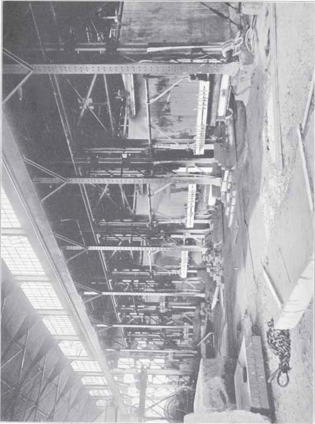
Installation of Six Bedford All Steel Gang Saws, Consolidated Stone Company, Bedford, Indiana
