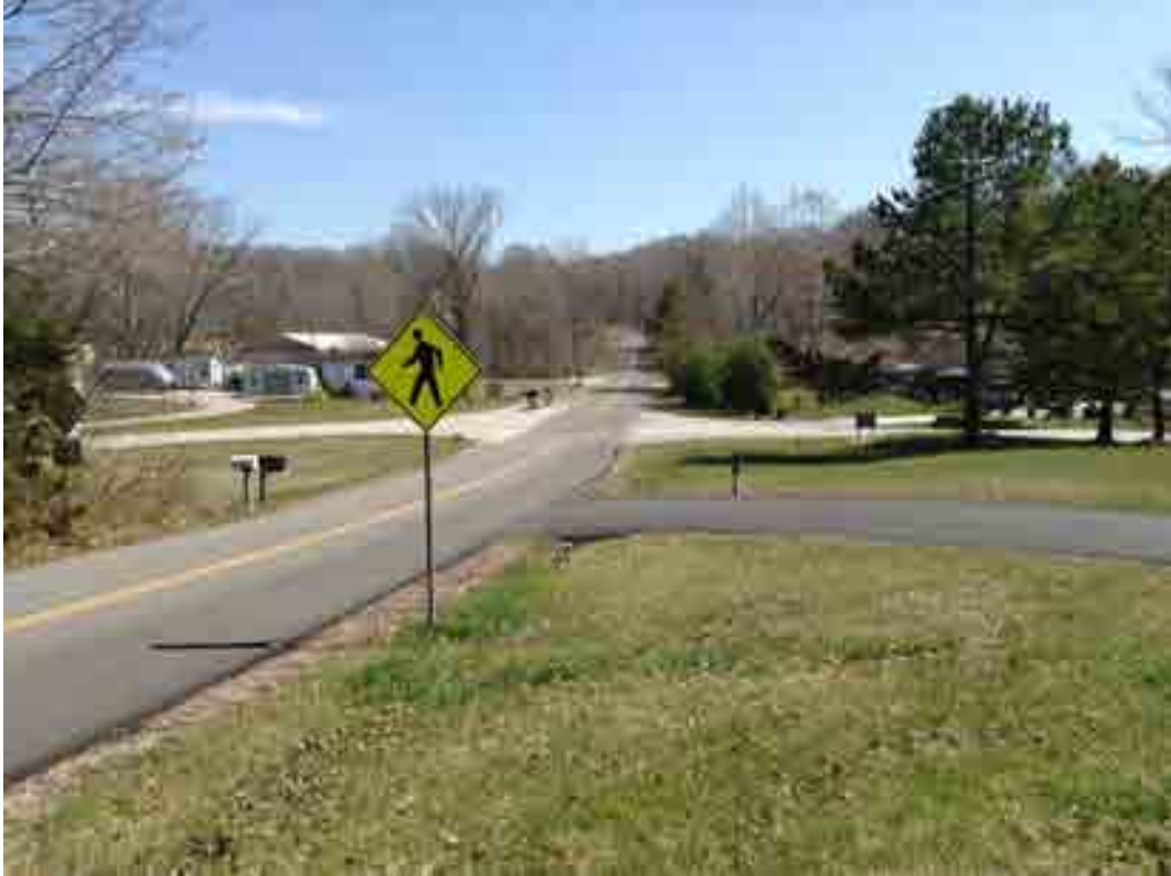
Photo 7 – Driveway cuts off E Northshore DR; facing southeast.
