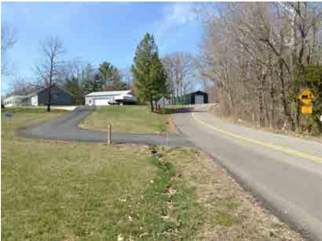
Photo 6 – 9550 & 9548 E Northshore DR driveway cut; facing northwest.
