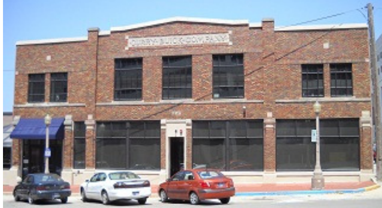
The Curry Building 214 West 7 th Street, Suite 200 Bloomington, Indiana 47404 (812) 349-2645
